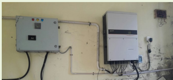
Fig. 5: Use of solar power panels in TU Campus
