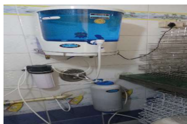
RO unit with demineraliser
